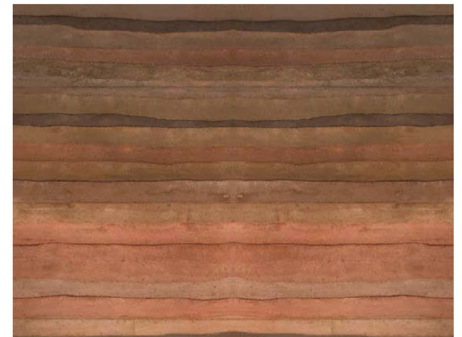
Using a mixture of earth and cement as the body
